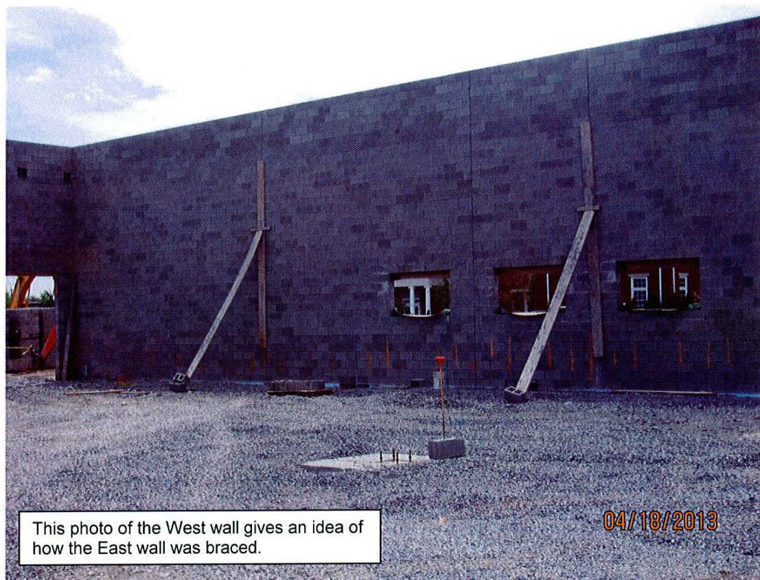
Photo 3. Interior wall bracing. (Photo courtesy of TOSHA.)
