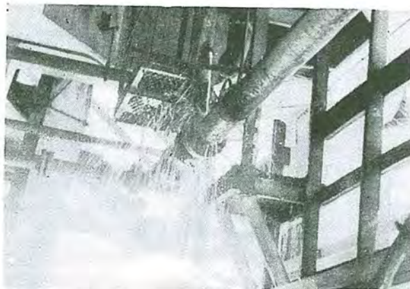
Figure 15. A leaking pipe, indicative of poor maintenance.
