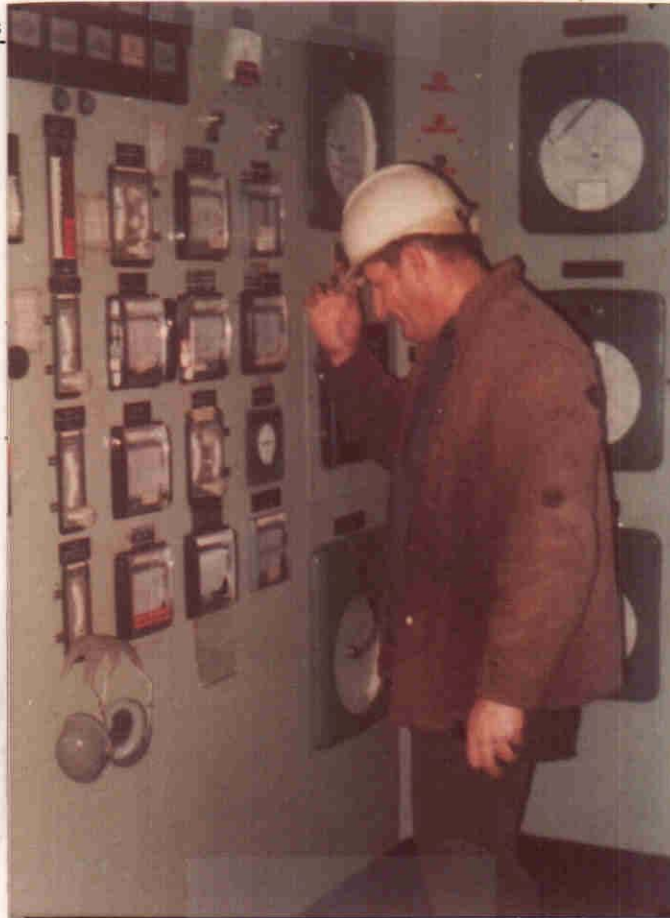
Monitoring mill telemetry instruments.
