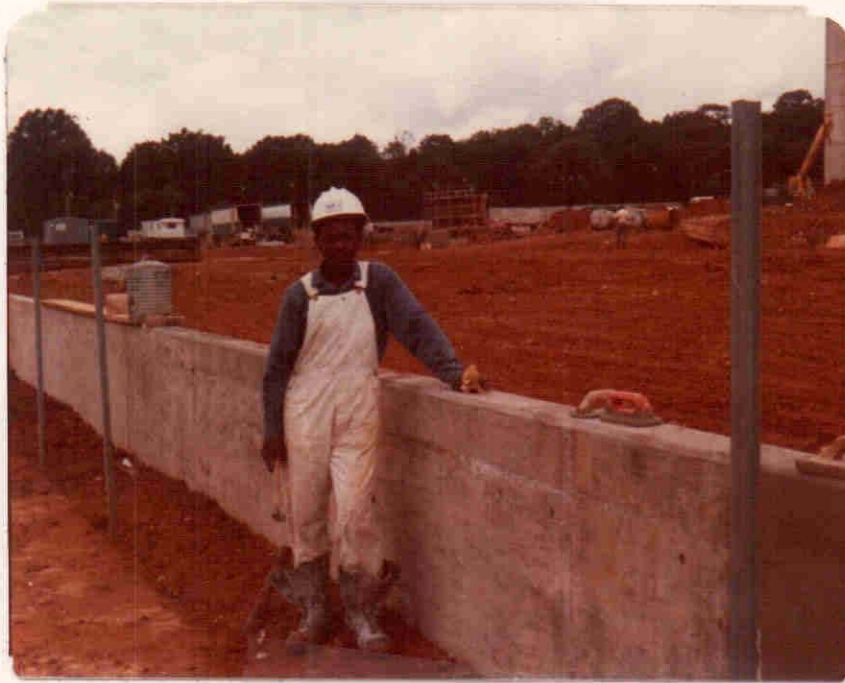
Mason finishing a cinder block wall.
