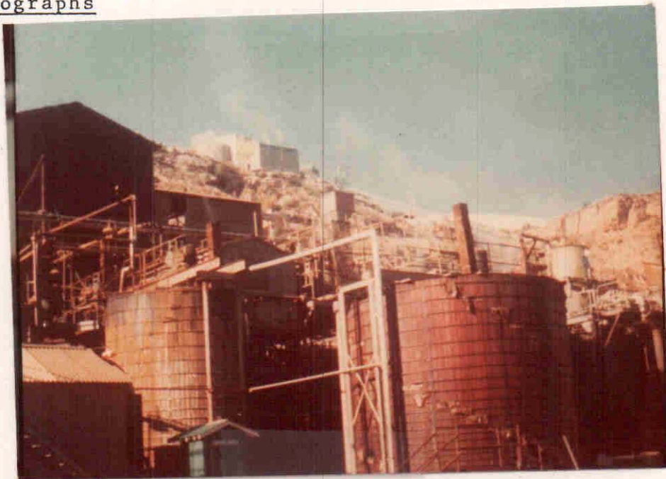
View of open ore slurry vats for vanadium processions.
