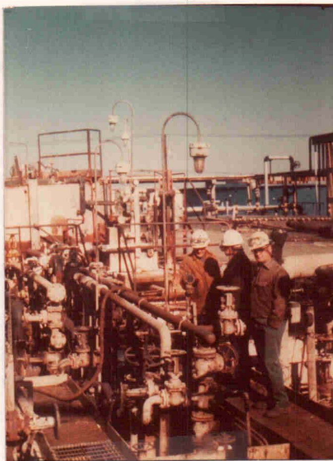
Refinery workers on structure changing defective valve.
