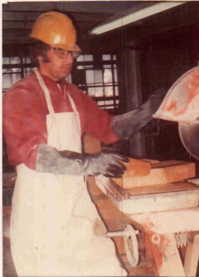
Employee cutting fire brick during furnace refurbishment
