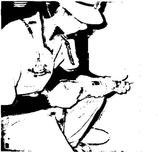
Figure 2. Fixing wall board to metal studs with screws by electric screw driver.
