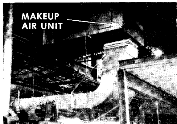
Figure 4-24. Tempered make-up air unit.
