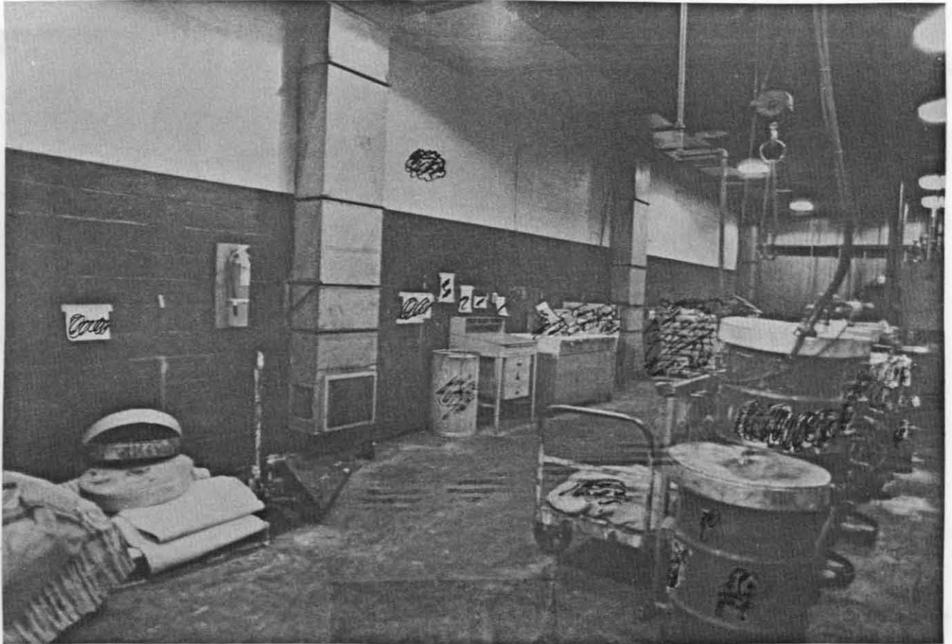
Figure 7-9. Cement house makeup air outlets. Note grills on front and sides. Also shown are palletted rubber and agitators.
