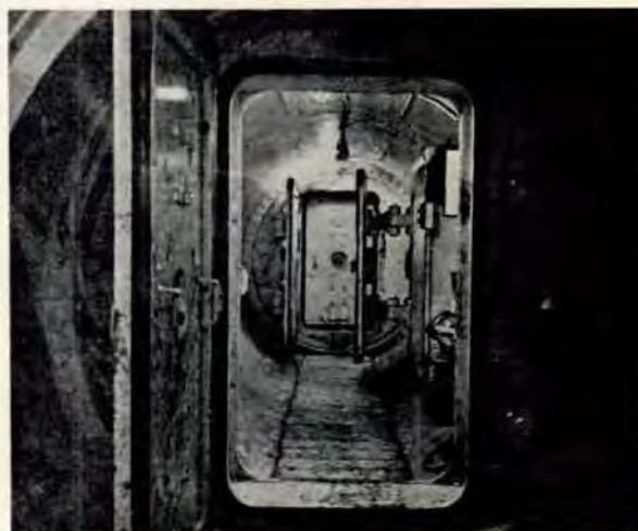
FIG. 4. Photograph of man-lock of 7½-ft diameter. Lock systems were automatically controlled by computer, which the lock tender set for the required decompression time. Highest pressure at which tunnel was operated, 36 psig, required decompression of 3 hr and 28 min. Door through bulkhead into compressed-air tunnel remained open at all times to allow miners to enter lock rapidly in case of emergency.
