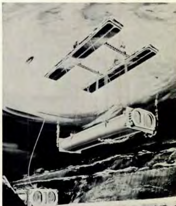
FIG. 1. Cable system used to lower tube sections from barge onto bottom of San Francisco Bay in course of Bay Area Rapid Transit construction. (Photograph courtesy of CIVIL ENGINEERING—ASCE, monthly publication of the American Society of Civil Engineers; September 1967.)
