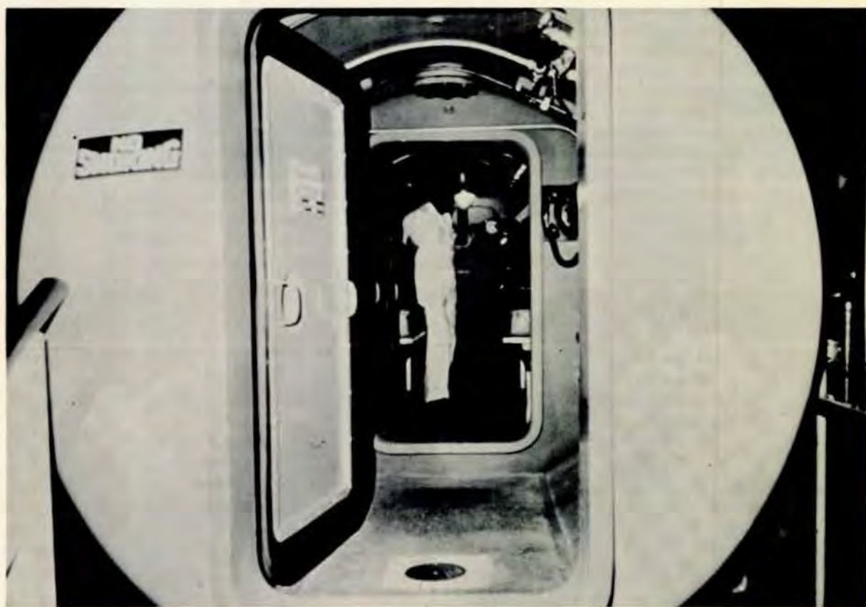
FIG. 5. Front and rear compartments of medical compression chamber at BART Transit Medical Center. Technician is standing inside inner treatment compartment.
