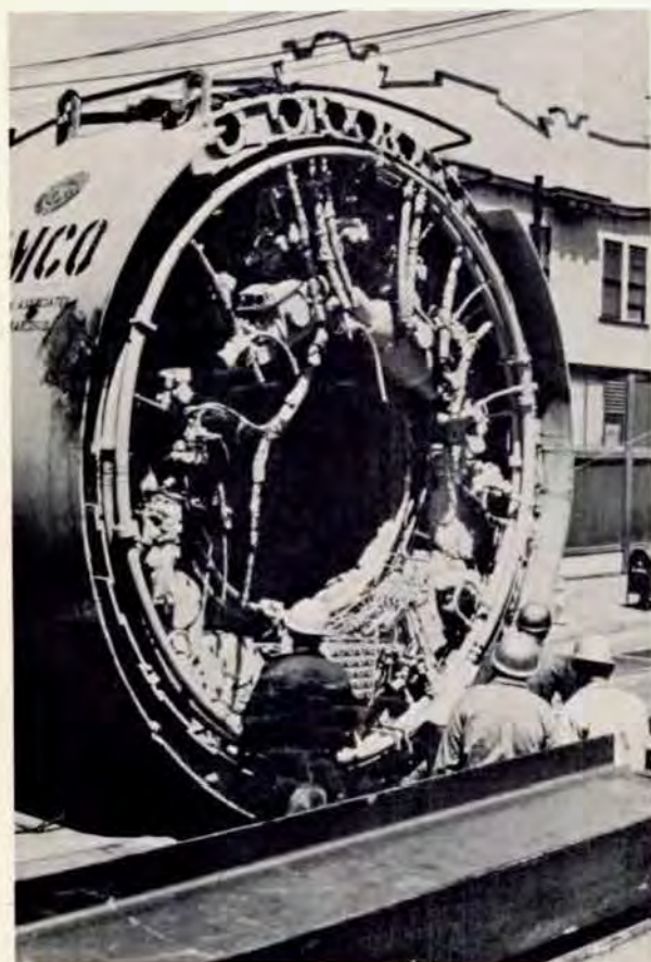
FIG. 3. Rear view of tunneling machine's cutting wheel, used in BART project.
