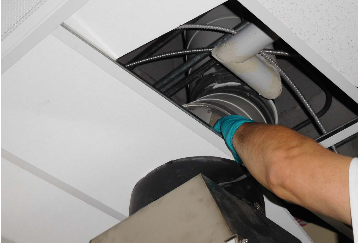
Figure 23. BSC exhaust (Photo Credit: NIOSH)
