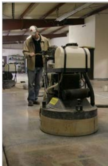
Figure 2: Floor polishing tool with water control (Courtesy of the Concrete Polishing Association)
