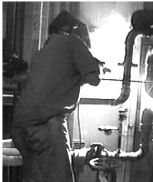
Figure 11. Worker Bending to Weld Pipe Onboard Vessel
