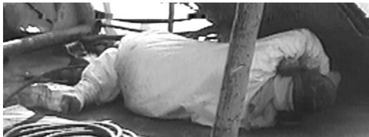
Figure 5. Deck Worker #2 Using Needle Gun
