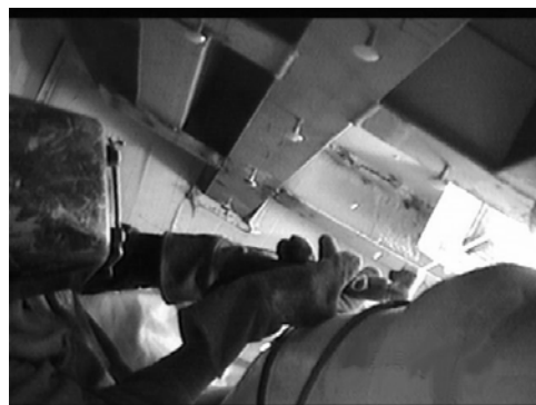
Figure 9. Welder Stick Welding Overhead
