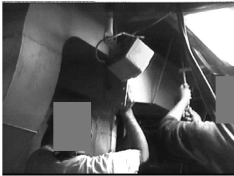
Figure 8. Duct Workers Lowering Duct from Overhead
