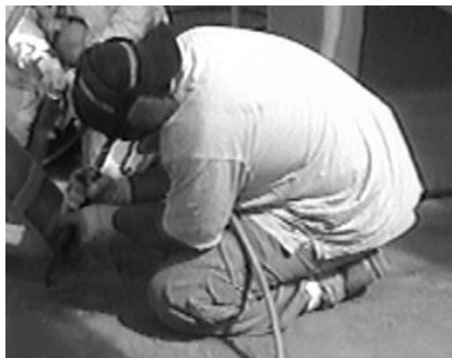
Figure 4. Deck Worker #1 Using Pneumatic Scraper
