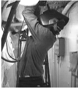
Figure 10. Worker Using Needle Gun Overhead
