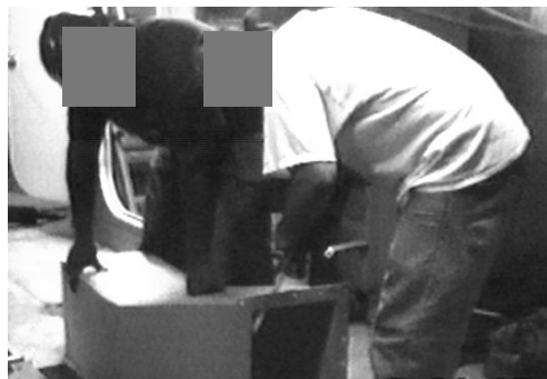
Figure 7. Duct Worker Cutting Flange
