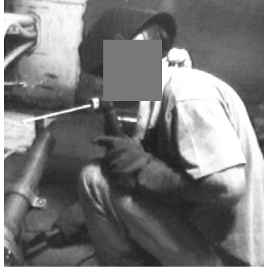
Figure 12. Worker Using Hammer to Deslag Pipe Weld
