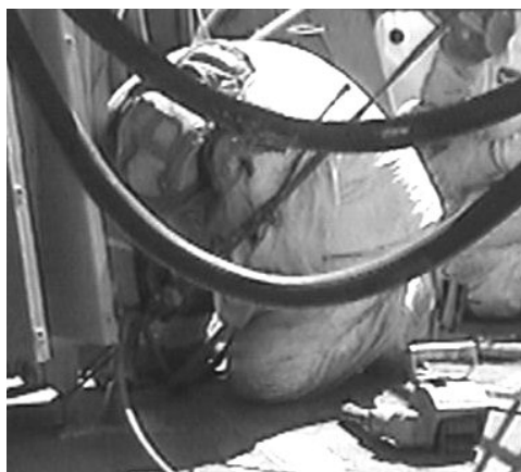
Figure 11. Deck Worker #2 Using Needle Gun
