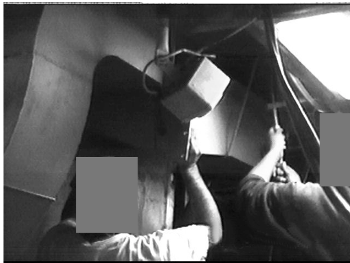
Figure 20. Duct Workers Lowering Duct from Overhead
