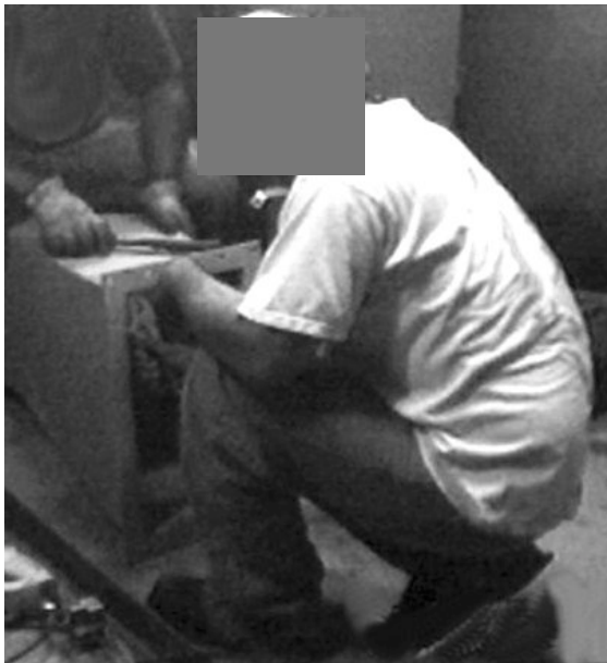
Figure 18. Duct Worker Removing Flange
