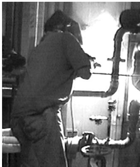
Figure 26. Worker Bending to Weld Pipe Onboard Vessel
