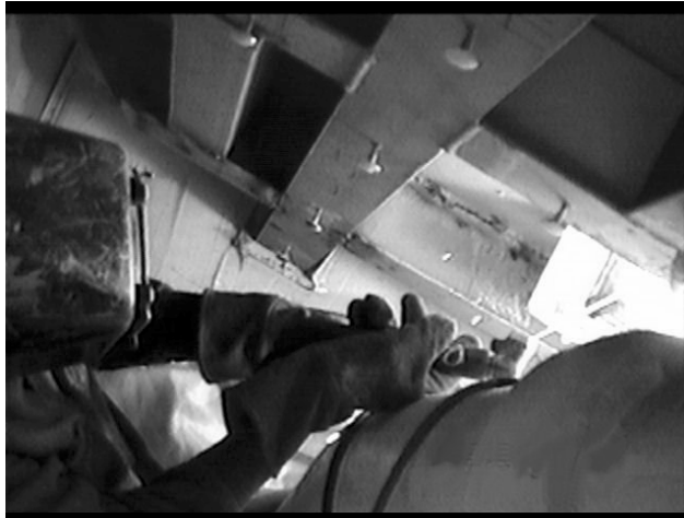
Figure 22. Welder Stick Welding Overhead
