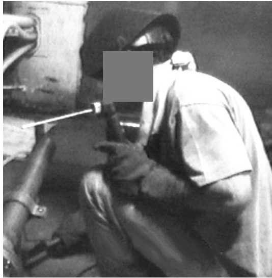
Figure 27. Worker Using Hammer to Deslag Pipe Weld
