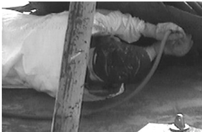
Figure 15. Deck Worker #3 Using Pneumatic Scraper
