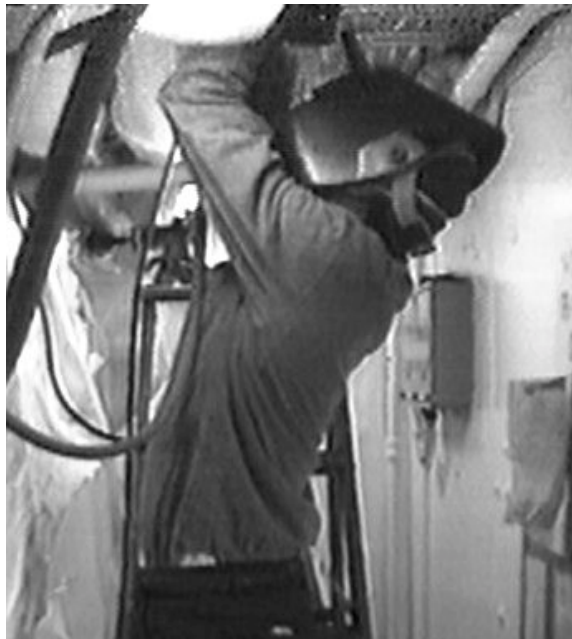
Figure 23. Worker Using Needle Gun Overhead
