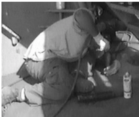
Figure 6. Deck Worker #1 Using Needle Gun
