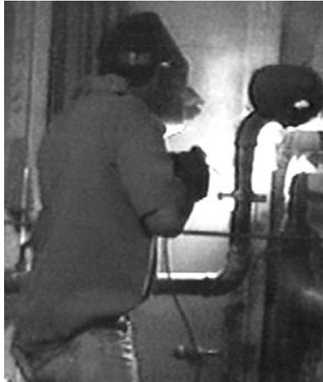
Figure 25. Worker Welding Pipe Onboard Vessel
