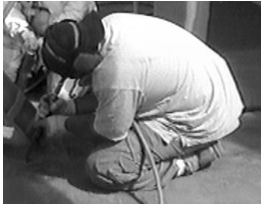
Figure 7. Deck Worker #1 Using Pneumatic Scraper
