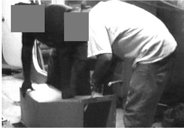
Figure 19. Duct Worker Cutting Flange
