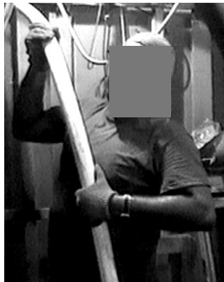
Figure 17. Cable Puller Holding 2-3" Diameter Cable, Waiting to Push -Up
