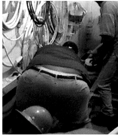
Figure 8. Cable Puller Squatting, Pulling 2-3" Diameter Cable Horizontally at Ankle Height
