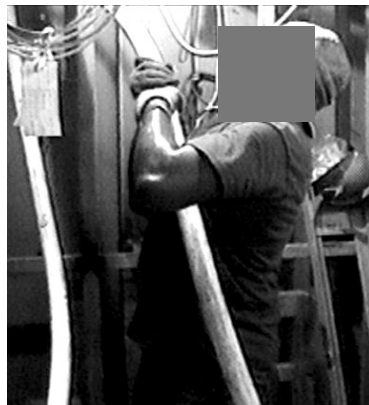
Figure 16. Cable Puller Pushing-Up 2-3" Diameter Cable, Body Extended Near End of Push
