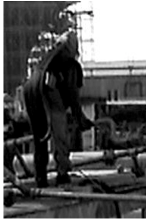
Figure 6. Abrasive Blaster Re-Positioning Material to be Blasted
