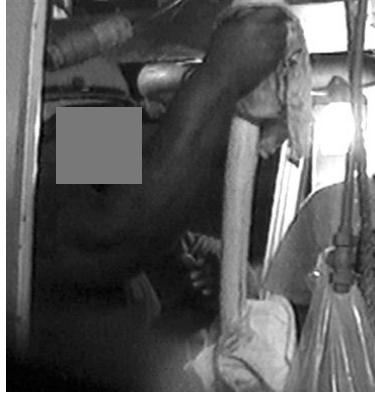
Figure 15. Cable Puller Holding 2-3" Diameter Cable Overhead, Tensed to Pull Down
