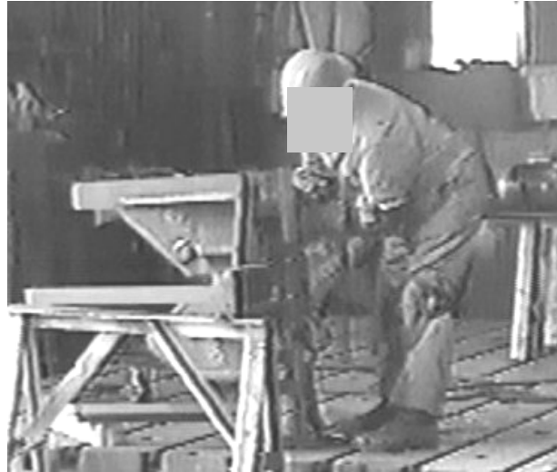
Figure 9. Tripod Welder Attaching Hoist Hook onto Subassembly
