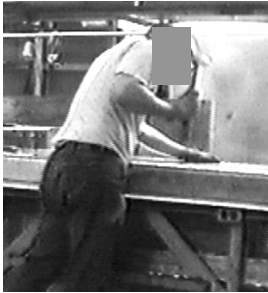
Figure 17. Sheet Metal Worker Hammering
