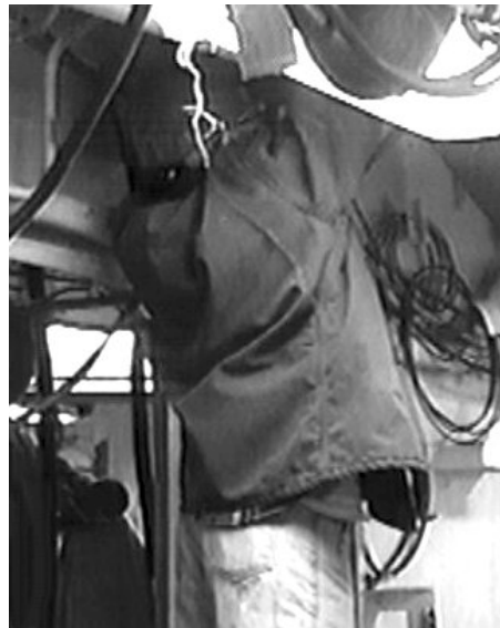
Figure 14. Cable Puller Standing, Tying Off 3/4" Diameter Cable Over Head
