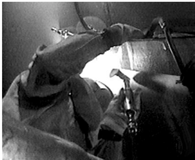
Figure 33. Tank Grinder Using 3 inch Offset Grinder
