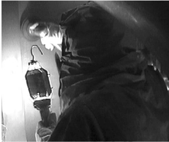
Figure 32. Tank Grinder Using 5 inch Offset Grinder
