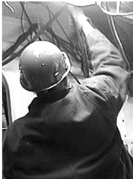
Figure 12. Cable Puller Standing, Feeding 3/4" Diameter Cable Over Head
