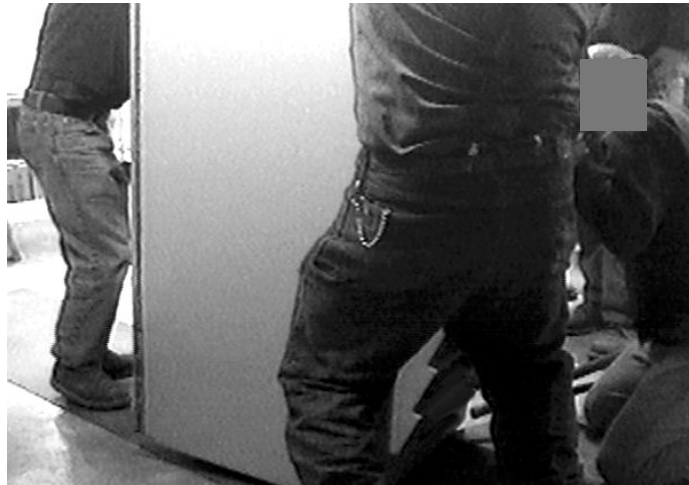
Figure 19. Tilting Equipment to Insert Pipe Rollers
