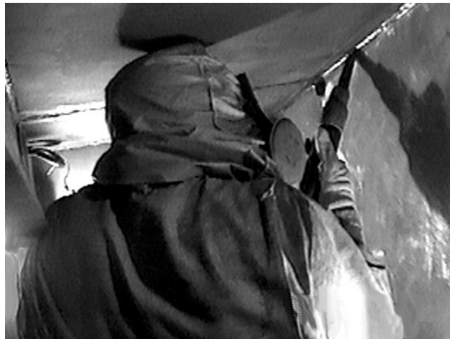
Figure 35. Tank Grinder Using Needle Gun Overhead
