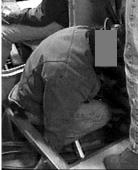
Figure 10. Cable Puller Squatting, Feeding 1.5" Diameter Cable Below Feet
