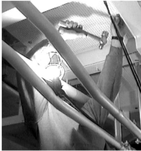
Figure 27. Insulation Installer Hammering Stud Caps Down
