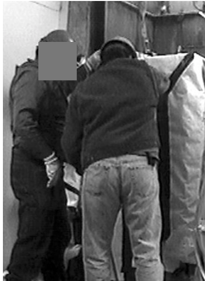
Figure 16. Rolling Equipment in on Low Profile Cart
