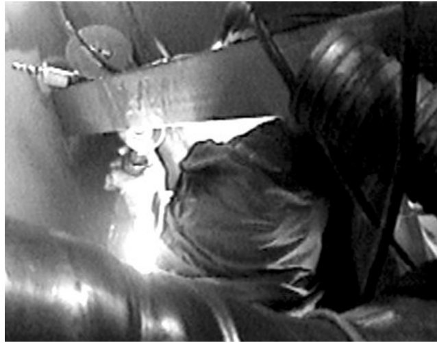
Figure 34. Tank Grinder Using Wire Brush
