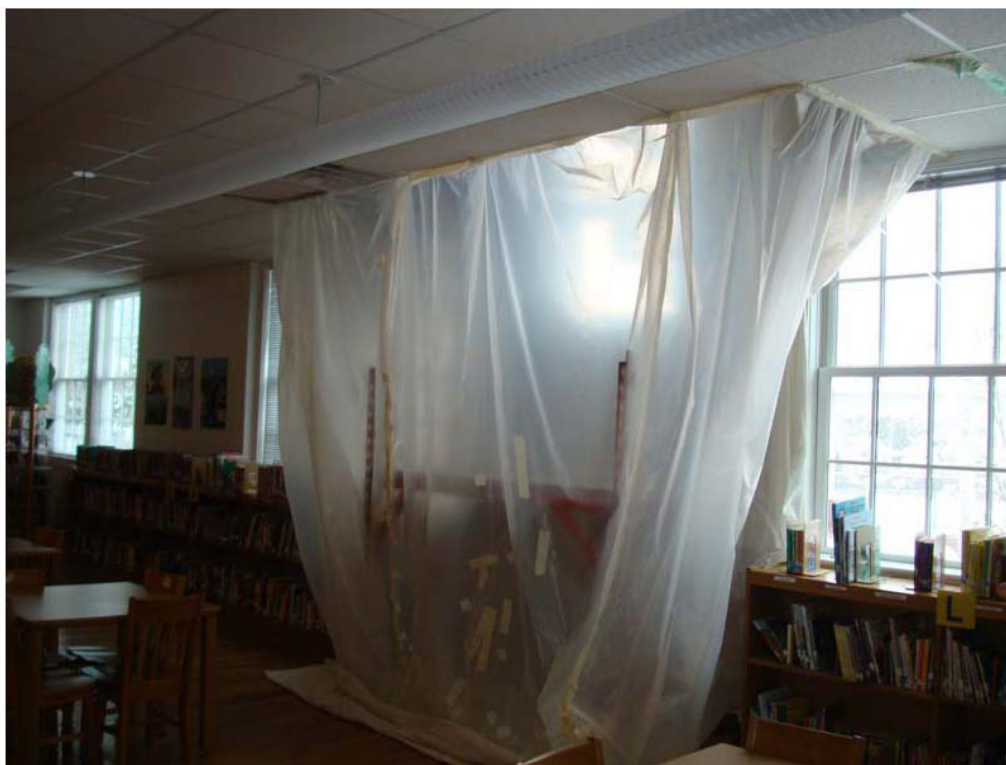
Figure 23. Media center, showing temporary containment barrier for installation of exterior door, March 2010.
