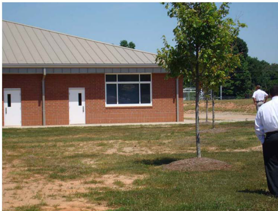
Figure 7. Downward sloping ground towards classroom wings, July 14, 2009
