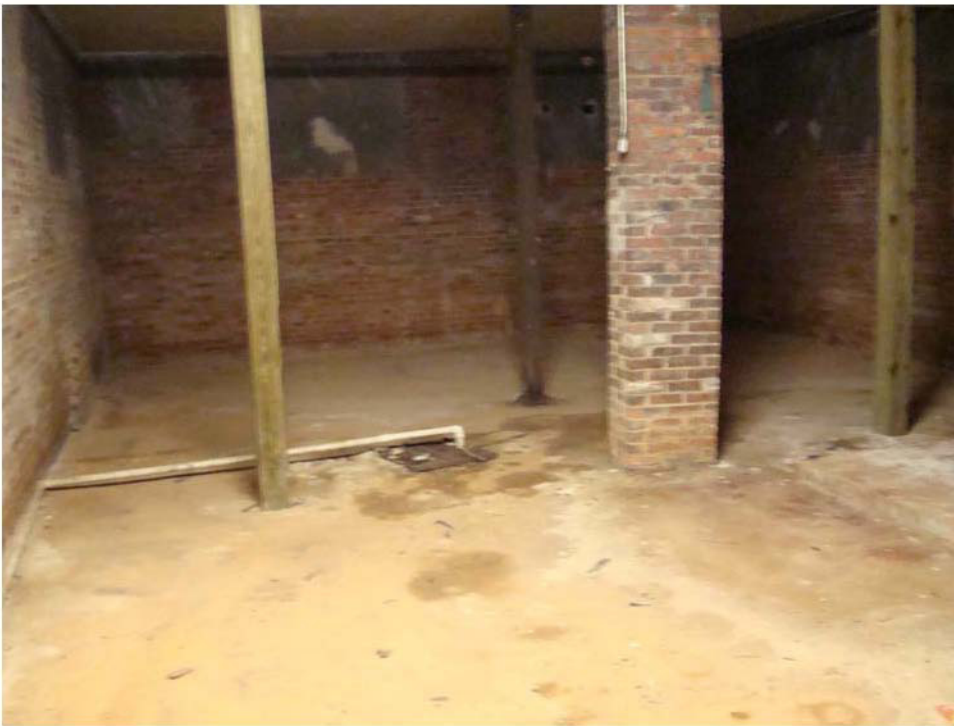
Figure 5. Basement below the media center wing, July 14, 2009
