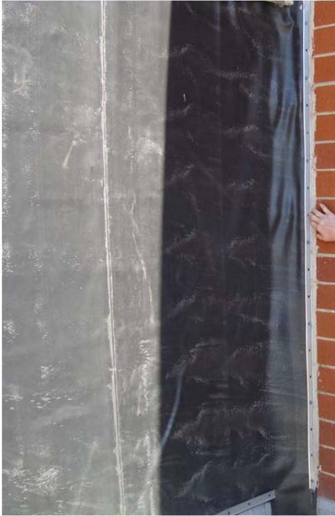
Figure 12. Inadequate flashing that appeared to be mounted superficially at the junction between the parapet wall (above room 206) and the gym, July 14, 2009
