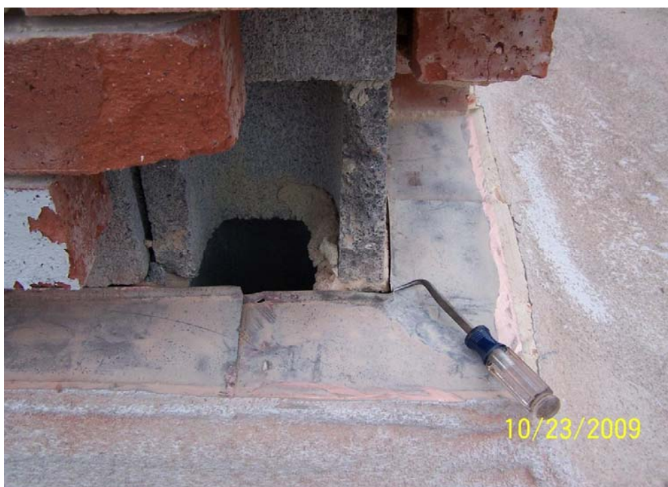
As Found Roof Flashing
