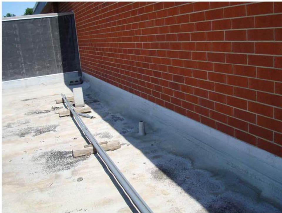
Figure 10. Foam roof adjacent to gym, July 2009.
