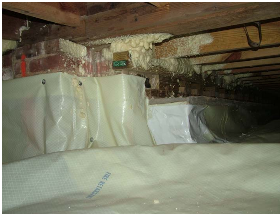
Crawl Space Vapor Barrier
