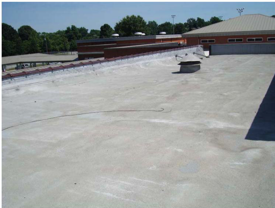
Figure 11. Foam roof over media center wing, July 2009.
