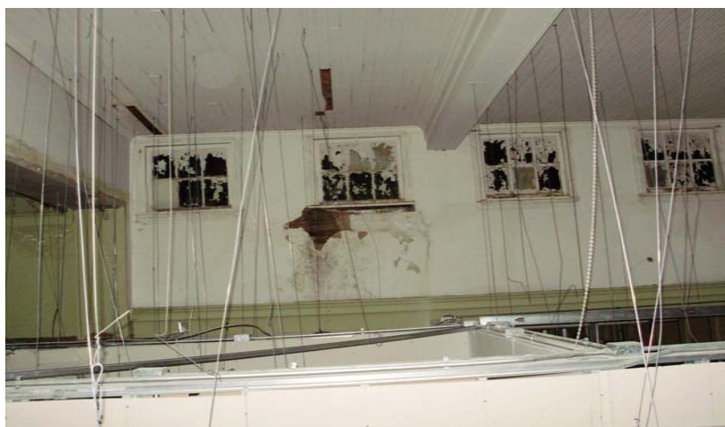
REMOVAL OF CEILING TILES
