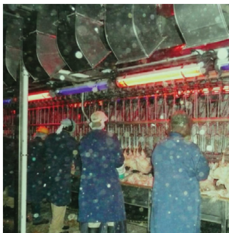
Figure 2. Employees in the live hang area. Supply air from ducts located above the employees' heads is directed toward the conveyor that is holding chickens to be shackled.
