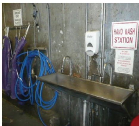
Figure 5. Hand washing station in the plant. The soap dispenser required the employee to push the lever to release the soap.
