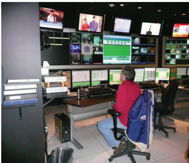
Figure 2. Employee surveying the fiber-optic fed video wall monitors (channel scan) and “thumbnail widgets” (split screens) on Barco branded screens in the VHO.
