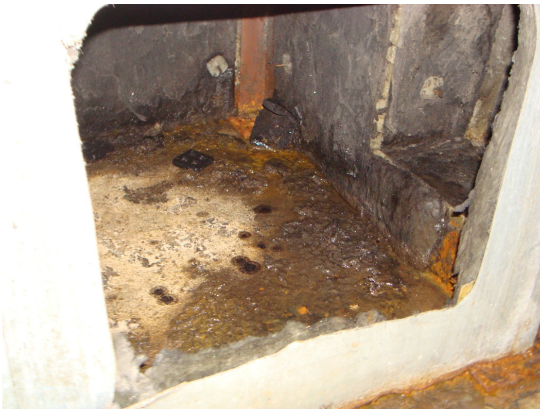
Figure 2. AHU-6 in the southeast corner mechanical room on the second floor of the shelter. The photograph shows condensate and debris in the return air plenum under the AHU.
