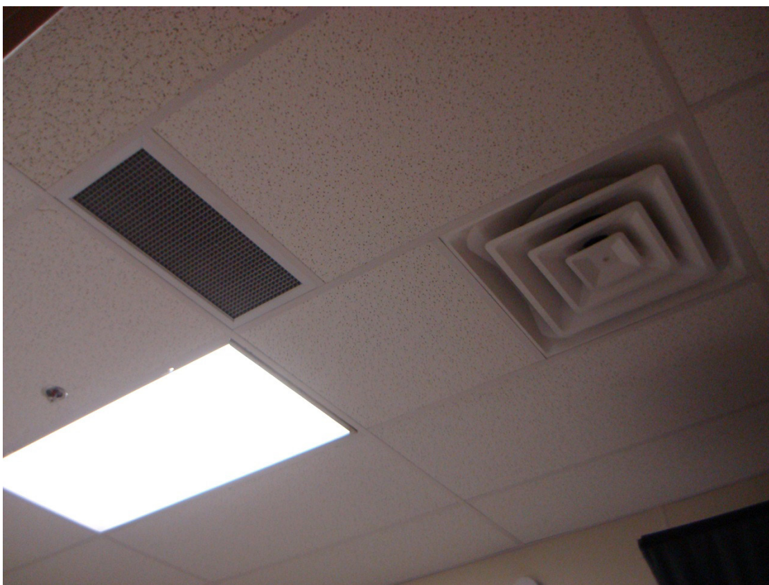
Figure 3. Supply vent and return grille in ceiling of family sleeping room #1 in the women's overnight facility. The close proximity of the supply to the return can result in short-circuiting of air, where supply air is immediately pulled into a return grille without providing any useful ventilation.
