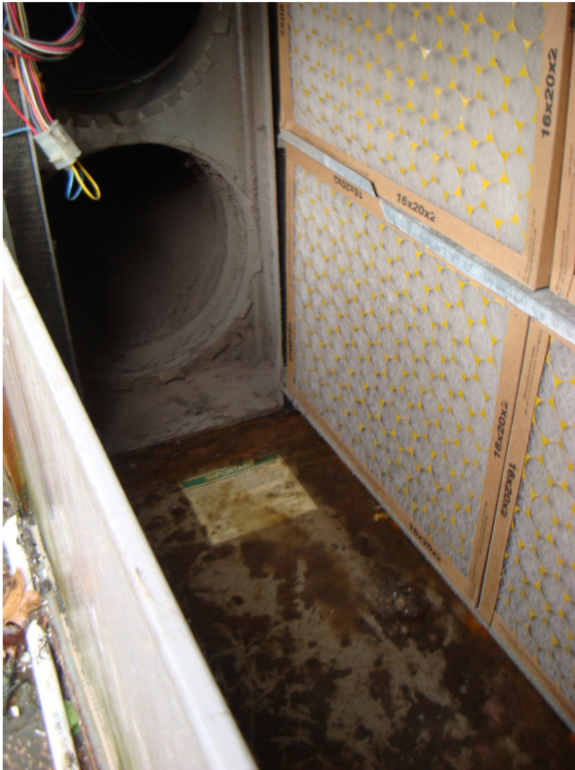
Figure 2. Standing water and apparent microbial growth in the drain pan of AHU Men-2.
