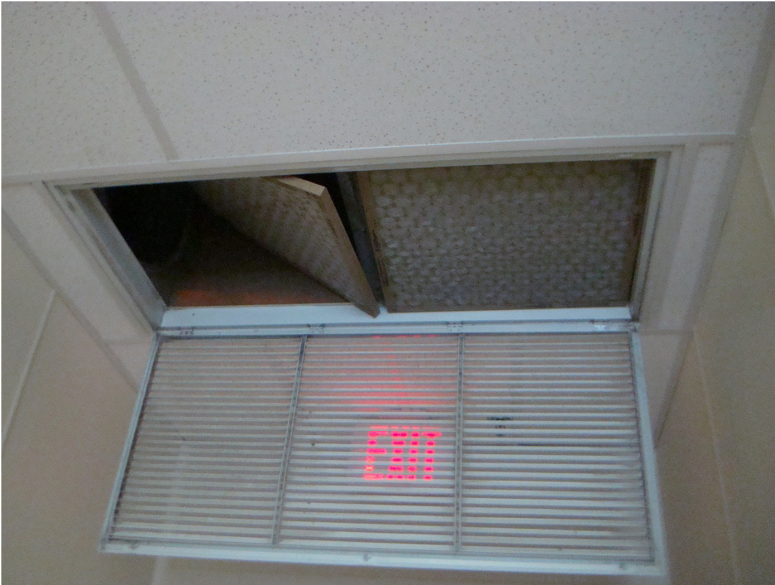
Figure 1. Return air grille leading to the AHU serving the women's overnight bunk area (Women-1). Air flow from the fan creates significant filter bypass.
