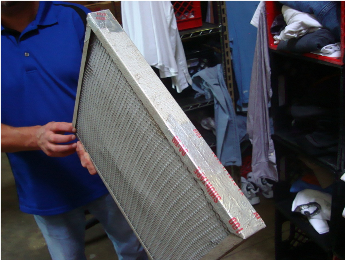
Figure 1. A representative ventilation filter from inside AHU Men-1, AHU Men -2, and AHU Men-4.
