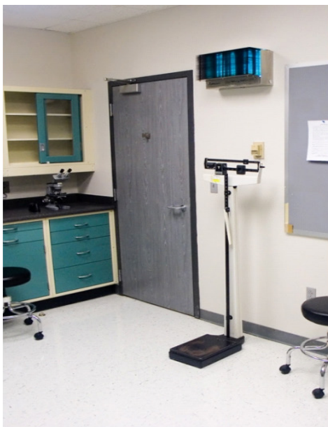
Figure 2. Typical upper-air UVGI installations: Left–Wall-mounted fixture with louvers installed in a health clinic; Right–Ceiling-mounted fixture with a fan installed in a homeless shelter.
