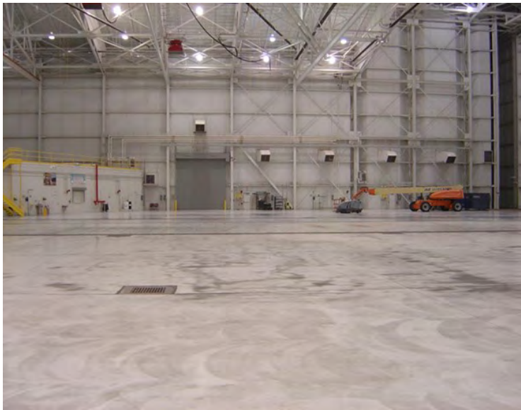
Figure 1. Photo showing location of air supply fans mounted on hangar wall. Photo by the National Institute for Occupational Safety and Health (NIOSH).
