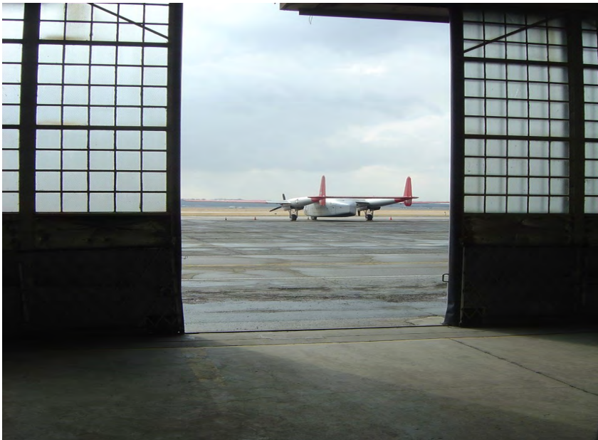
Figure 6. Photo of restoration hangar front bay doors that were opened to provide some supply air. Photo by NIOSH.
