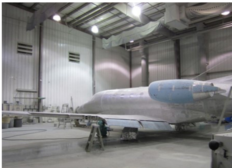
Figure 9. An aircraft parked in the stripping bay. Outdoor air was provided by a ceiling-mounted air handler and distributed through perforated, flexible plastic ducts (top right). Conditioned air was supplied through two wall fans in front of aircraft. The location of outdoor and conditioned air supplies created turbulence and reduced the effectiveness of the floor mounted exhaust ventilation system. Photo by NIOSH.
