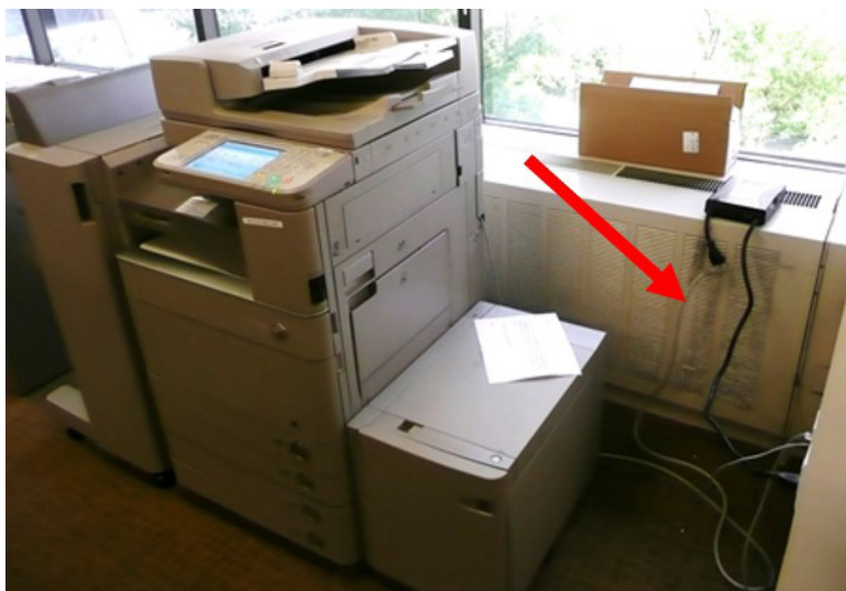
Figure 2. A laser printer located next to the air intake of the nearby peripheral fan-coil unit. The arrow points to a section of the air intake that is likely discolored by the printer's emissions. Photo by NIOSH.
