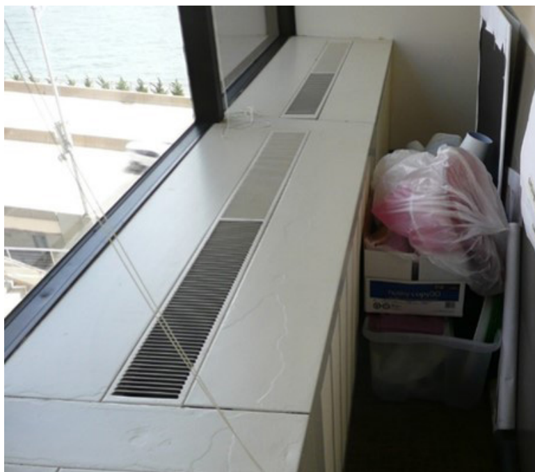
Figure 1. Office supplies and boxes blocking the air intake of a peripheral fan-coil unit. Photo by NIOSH.
