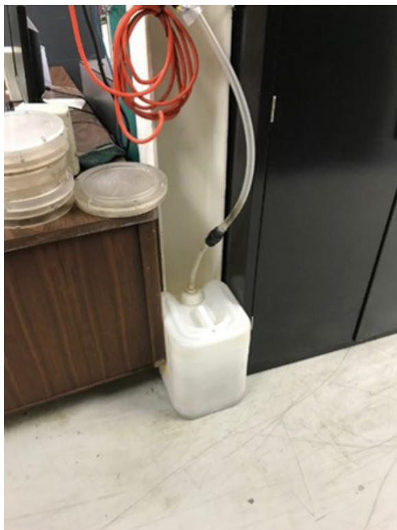
Figure 2. Catch basin that is connected to the ductwork between the molding and printing departments. There is a hose running up the wall connecting to the ductwork between the molding and printing departments (ductwork not pictured). Photo by NIOSH.
