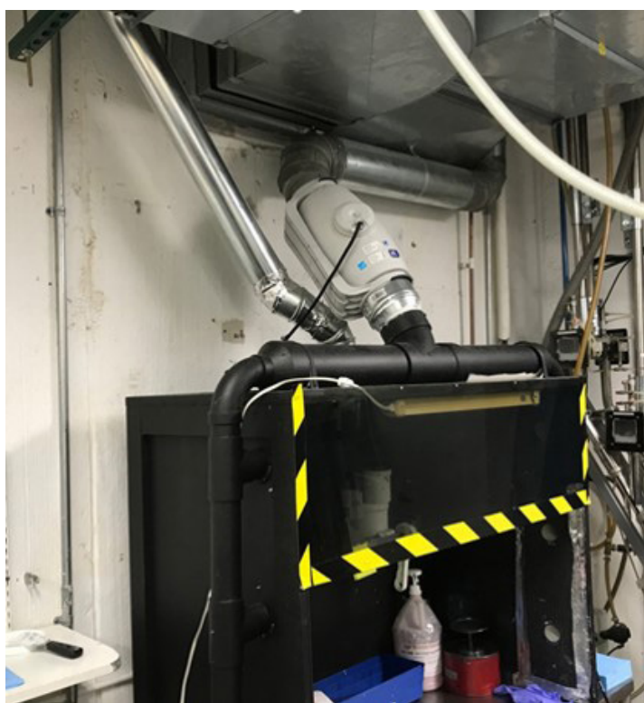
Figure 1. Photograph of the handmade hood in the printing department. Screen wash is dispensed from the red plunger can inside the hood, and the sash is not adjustable. Photo by NIOSH.
