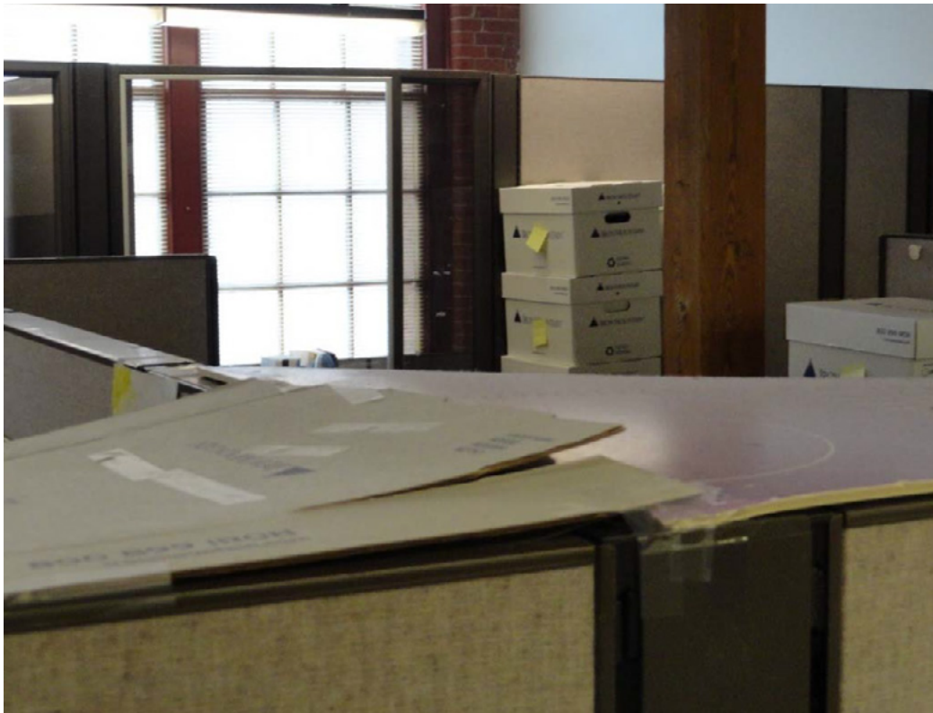
Figure B3. Personal workspaces partially covered with poster board to block dust from heating, ventilation, and air-conditioning system at an office building on June 1, 2018. Photo by NIOSH.
