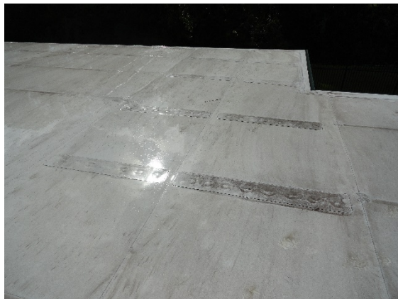
Figure 9. Patching on roof. Photo by NIOSH.
