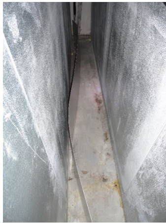
Figure 4. Visible water damage/stains between the walk-in freezer and refrigerator in the evidence area. Photo by NIOSH.
