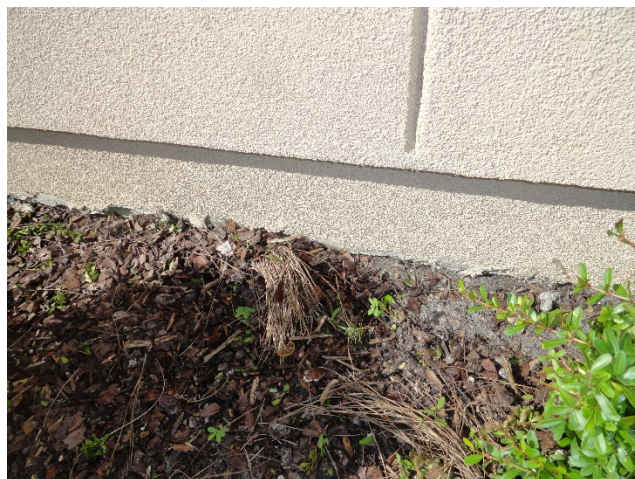
Figure 10. Exposed cement block near the base of exterior wall. Photo by NIOSH.
