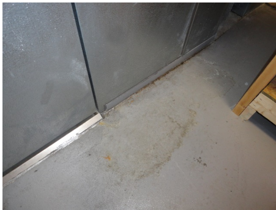
Figure 3. Visible water damage/stains in front of the walk-in refrigerator in evidence area. Photo by NIOSH.
