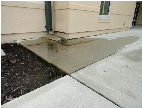
Figure 7. Water pooling in mulch and against building from downspout at front of building. Photo by NIOSH.
