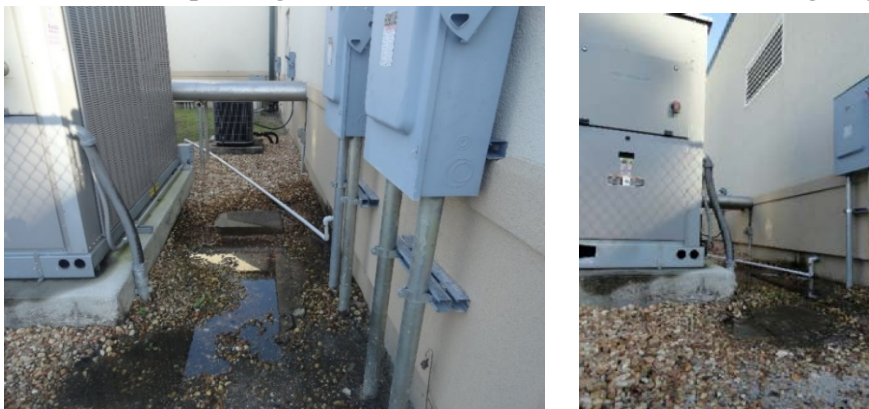
Figure 6. Water pooling under fresh air intake near the emergency generator. Photos by NIOSH.
