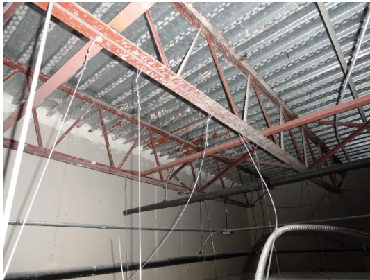
Figure 2. Rust on metal roof above the ceiling tiles in room 129. Photo by NIOSH.
