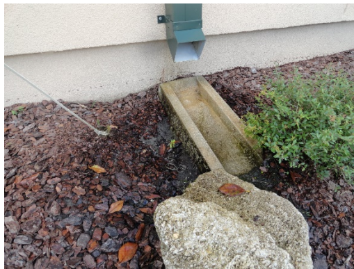
Figure 8. Water pooling in mulch and against building near outdoor patio space. Photo by NIOSH.
