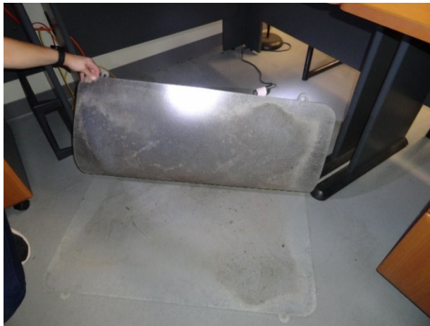
Figure 5. Visible stains and mold odor under plastic mat on concrete floor in the evidence room. Photo by NIOSH.
