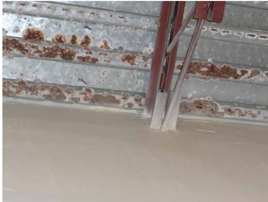
Figure 1. Rust on ceiling in the evidence room. Photo by NIOSH.
