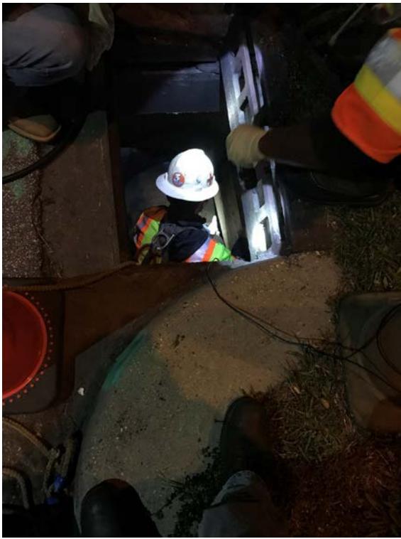
Figure A6. Employee cutting water-cured liner inside of access hole at CIPP installation, March 2019. Photo by NIOSH.
