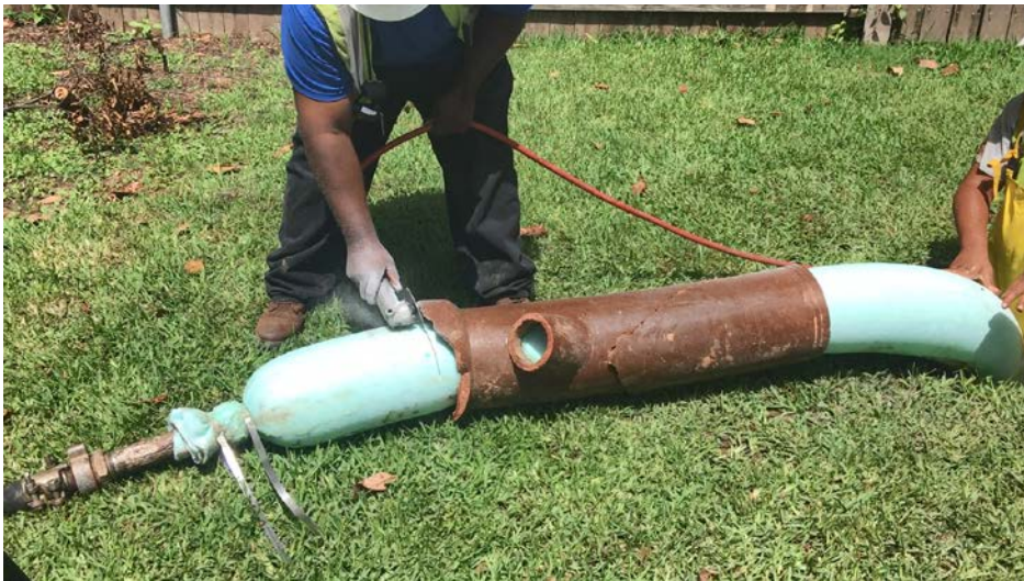
Figure A8. Employee cutting excess section of steam-cured liner outside of manhole at CIPP installation, June 2019. Photo by NIOSH.
