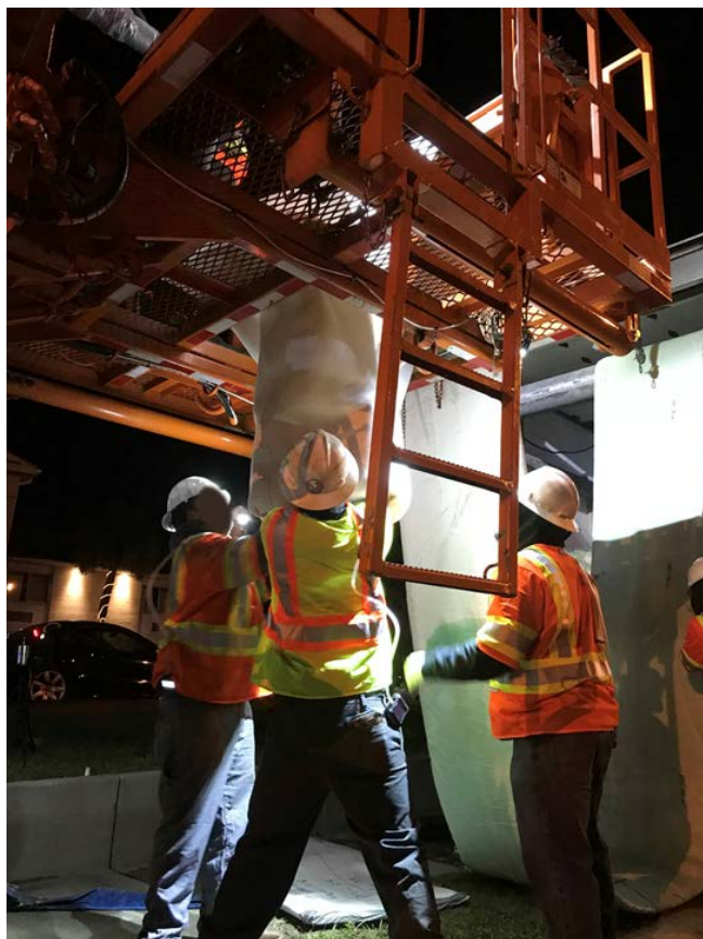
Figure A5. Employees pulling dry liner through itself under lift on boiler truck during water-cured CIPP installation, March 2019. Photo by NIOSH.
