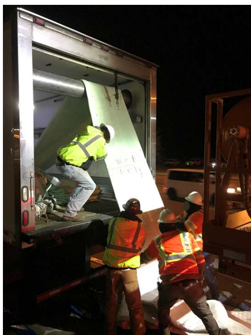
Figure A4. Employees removing liner from refrigerated truck during water-cured CIPP installation, March 2019. Photo by NIOSH.
