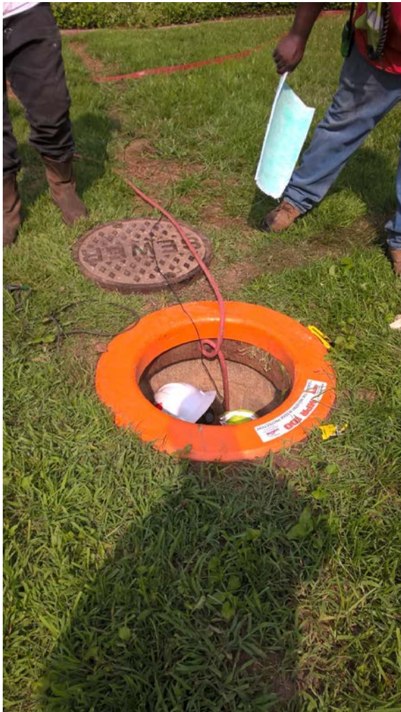
Figure A9. Employee cutting steam-cured liner fully inside of manhole at CIPP installation, June 2019. Photo by NIOSH.
