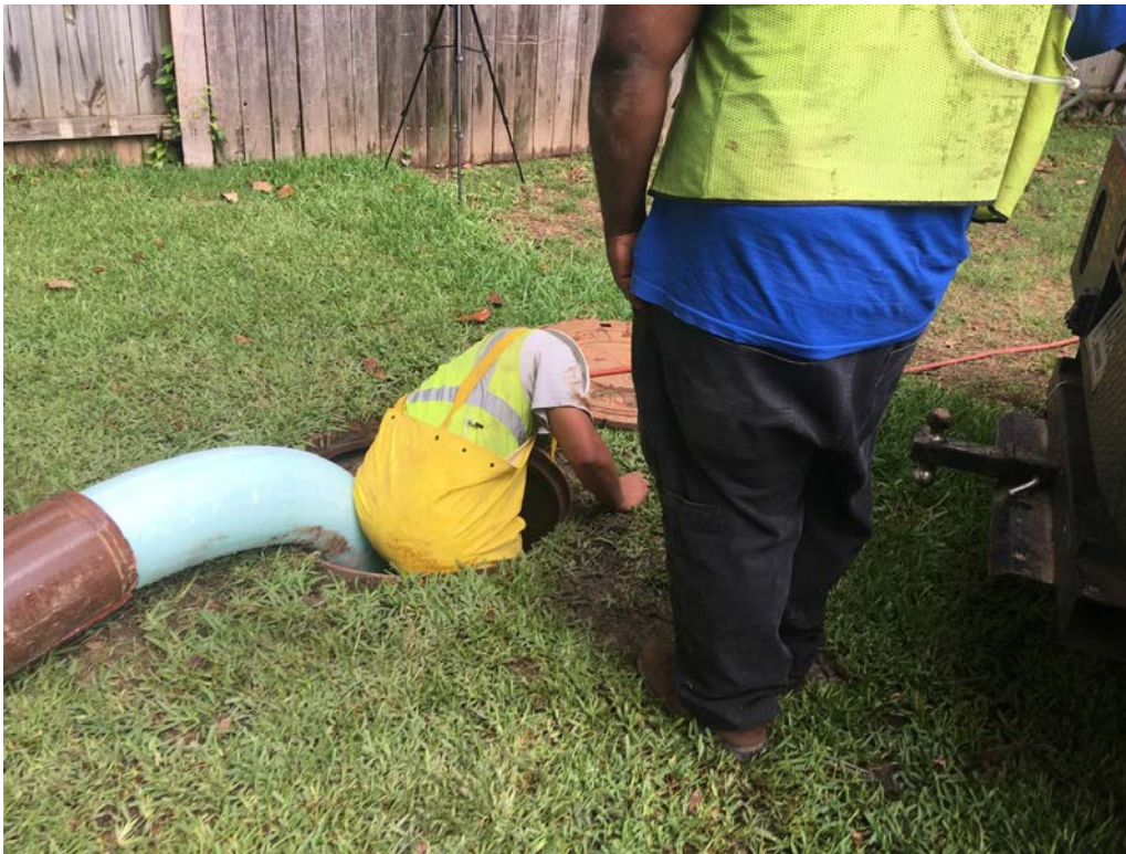
Figure A7. Employee cutting steam-cured liner partially inside of manhole at CIPP installation, June 2019. Photo by NIOSH.
