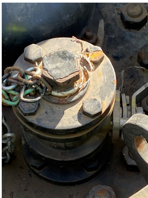
Figure B9. Valve inside the housing with a damaged seal on the valve cover. Photo by NIOSH.
