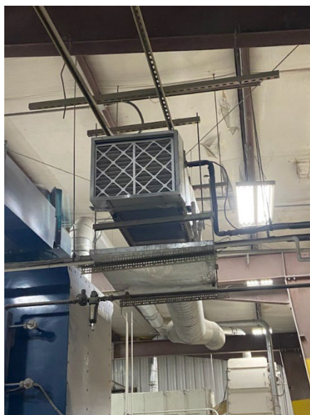
Figure B2. Air intake through a pleated filter, air-conditioner, and supply ductwork for one of the two air conditioning units in the lamp room. Photo by NIOSH.
