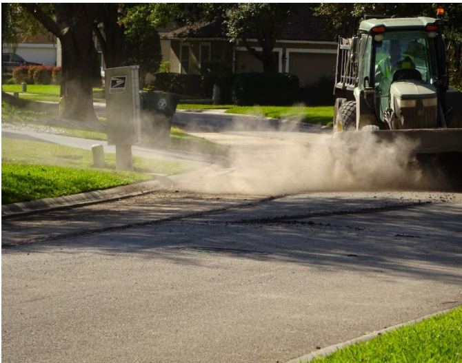
Figure A12. Dry sweeping road with rotary broom after asphalt milling prior to re-paving. Photo by NIOSH.
