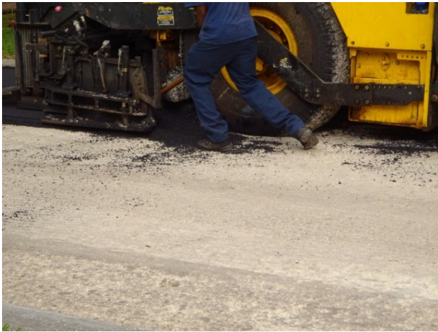
Figure A14. Paver/screeder machine laying down asphalt over freshly-milled road surface. No observable dust generated during this task. Photo by NIOSH.
