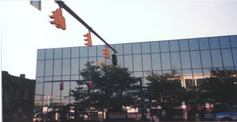
Front View of Building Accident Occurred
