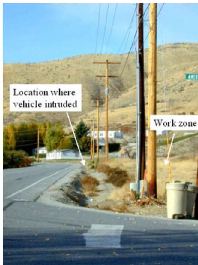
Photograph 3. The location of the work zone, after the incident.
