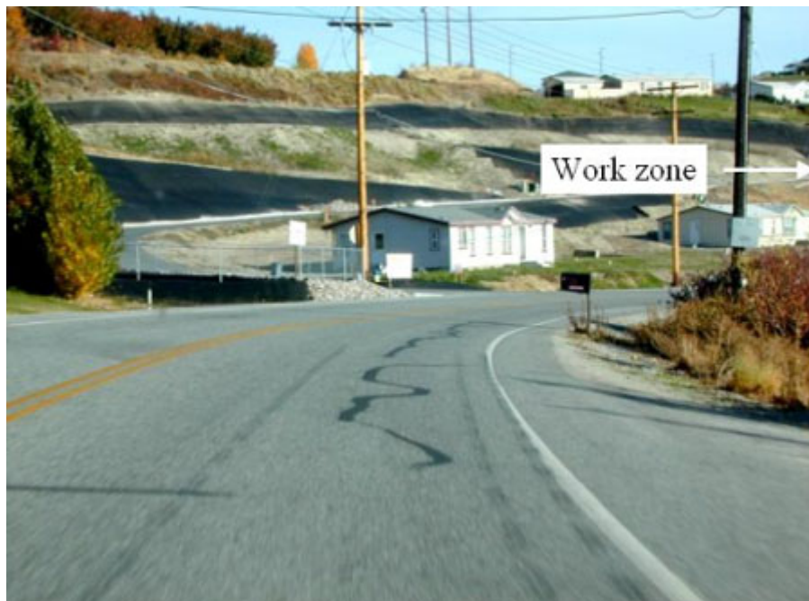
Photograph 1. View approaching the work zone from the south (direction from which the intruding vehicle approached).
