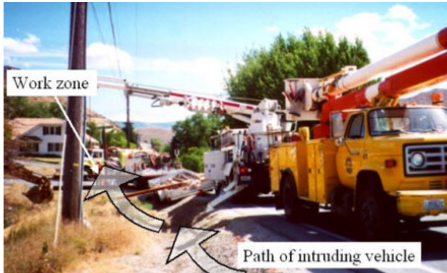
Photograph 2. The work zone.
