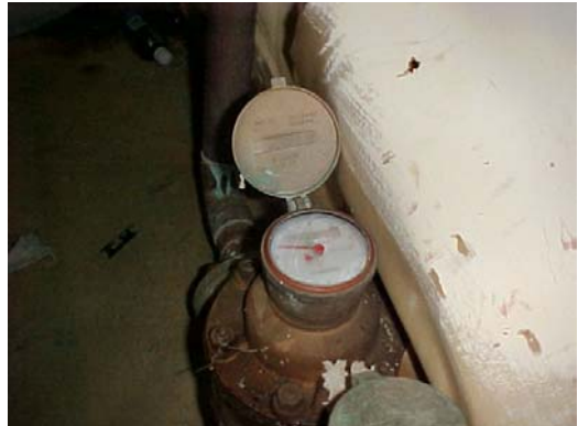
Figure 2. Water meter at floor level
