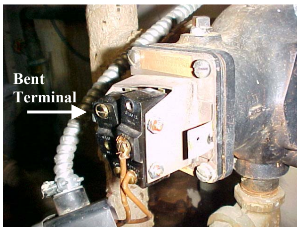
Figure 4. Low water switch terminals after victim contact
