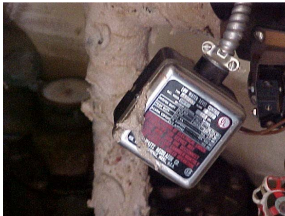
Figure 3. Low water switch box cover hanging from bracket
