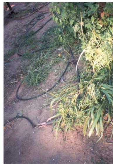
Figure 4. Un-insulated splice
