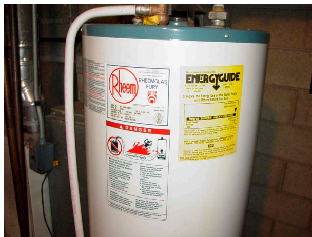
Figure 3. Location of flammable material warning label on side near top of heater
