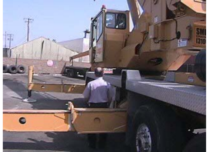
Exhibit 4. A simulated picture depicting the victim's position while the crane rotated into position.
