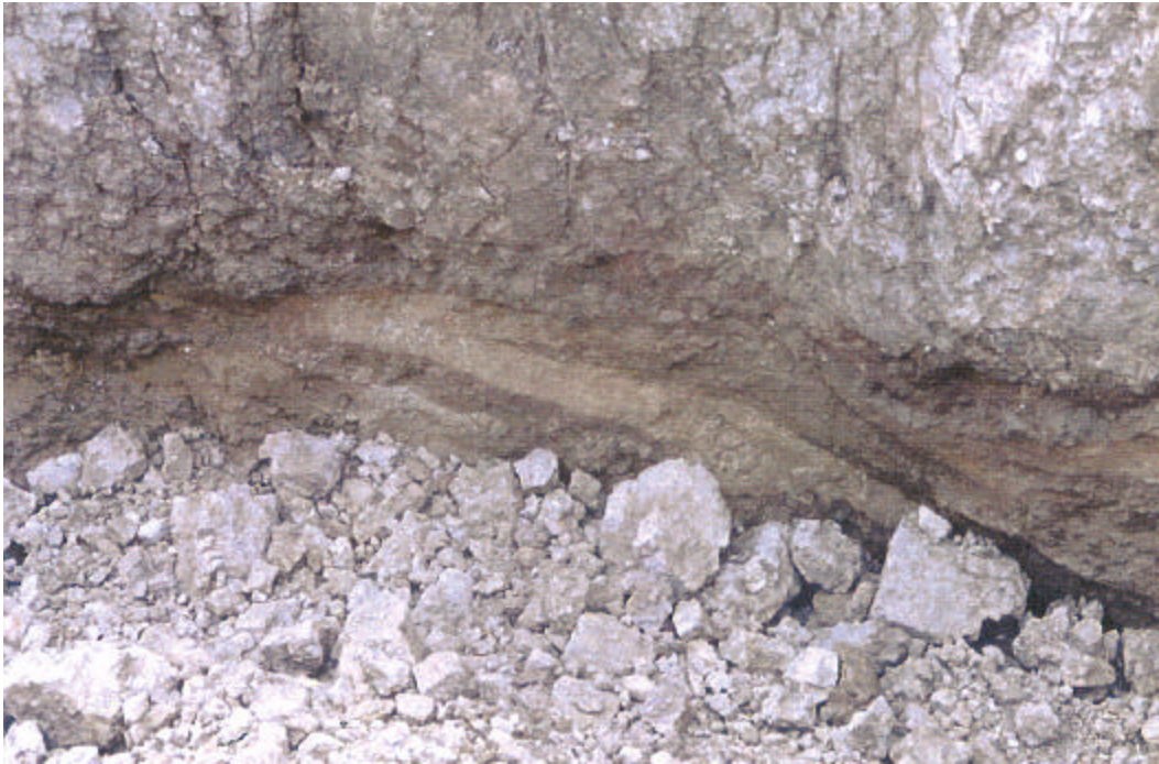
Figure 3. Cave-In Area (Looking South, cave-in area is approximately 30 feet long and 11 to 13 feet deep.)
