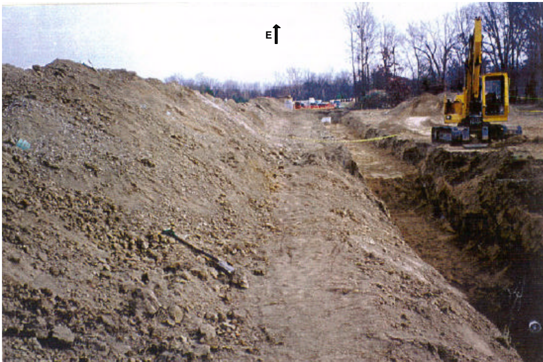
Figure 1. Sewer Installation Project (Trench pictured is approximately 200 feet long.)
