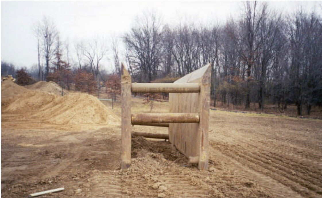
Figure 2. Shield (Shield was removed from the trench with an excavator and placed 20 yards from the trench.)
