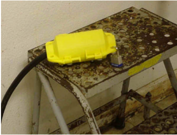
Photo 5. Typical Method of Locking Out Line Cord Plug
