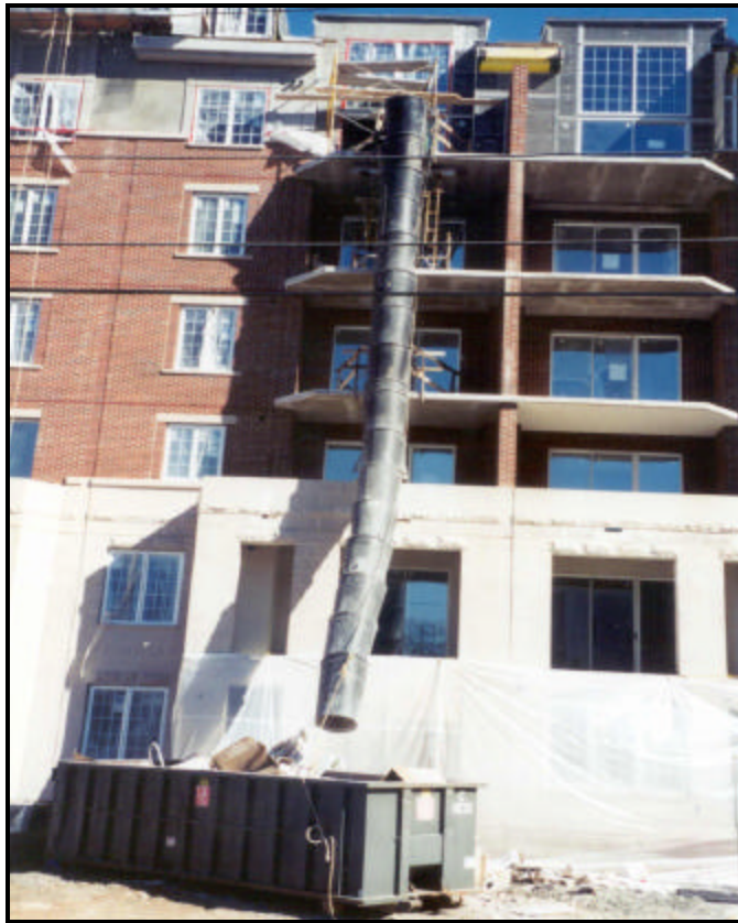
Photo 1. This photo illustrates the debris chute on the building where the incident occurred. The photo was taken 1 month following the incident: an additional structure had been built in front of the window that the victim and coworkers were attempting to cover
