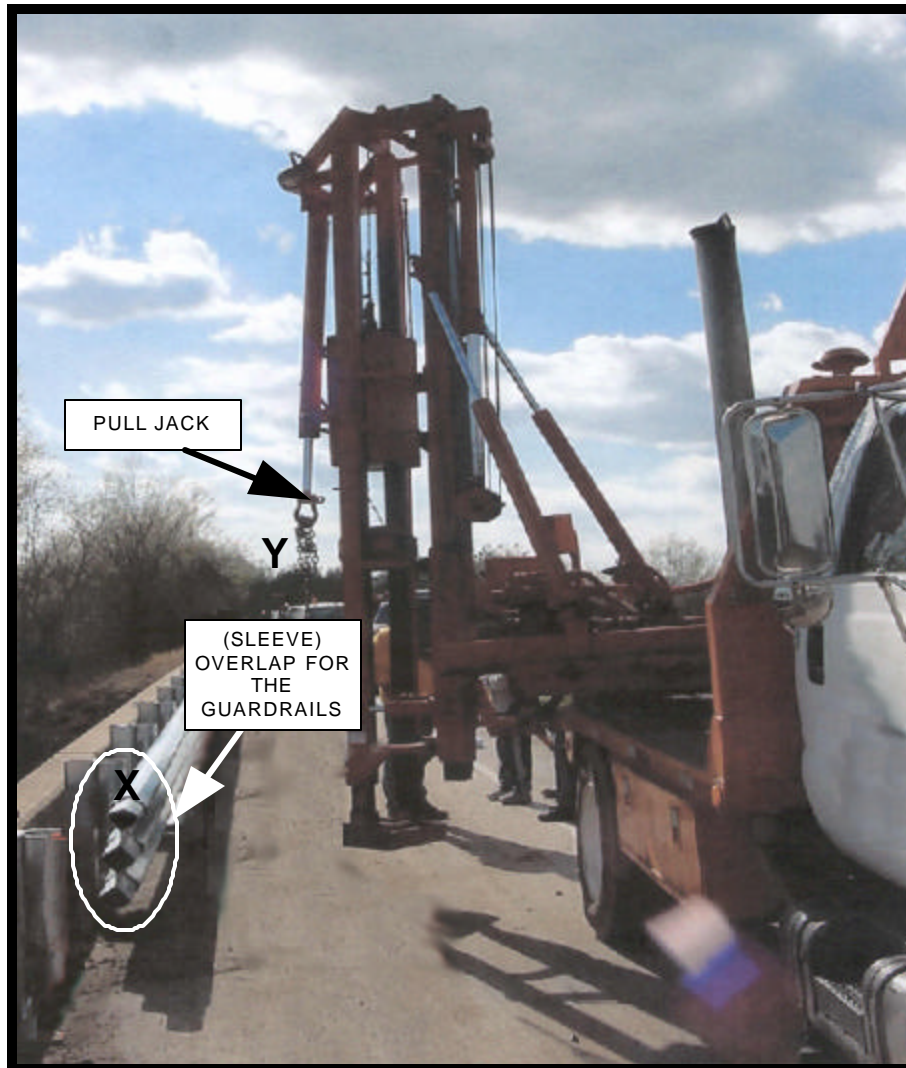
Photo 1. This photo illustrates the truck-mounted post driver used on the day of the incident. An "X" marks the installed section of guardrail. The section of guardrail being lowered was to be slid onto the existing guardrail, like a sleeve. A "Y" marks the pull jack of the post driver. Photograph courtesy of the County Sheriff's Department.
