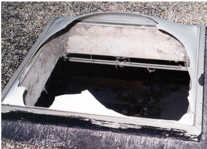
Photo 2: This photograph illustrates a close-up taken from the roof of the skylight through which the victim fell.
