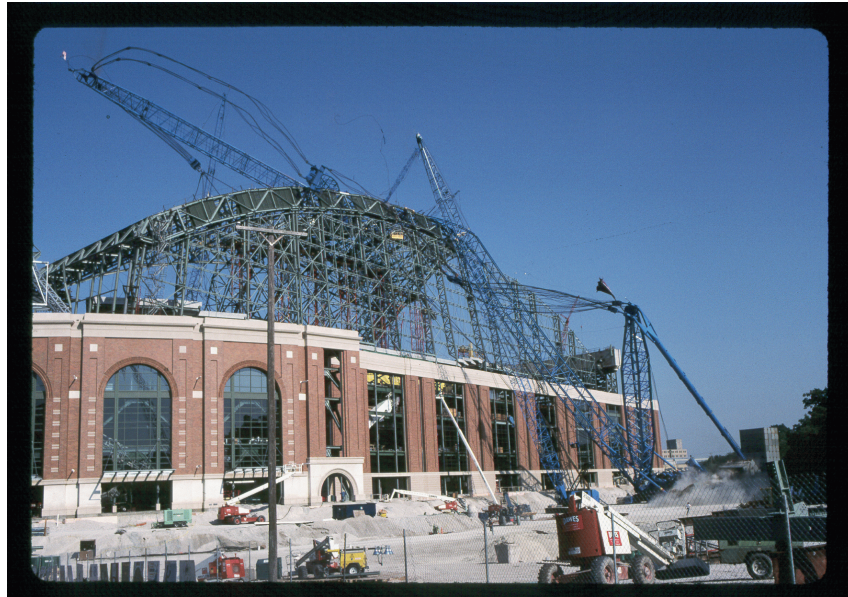
Photo 1: Heavy-lift crane during tipover at stadium (Photo courtesy of John A. Thraen)
