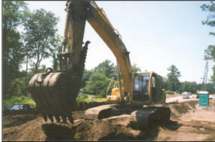
Excavator involved in incident
