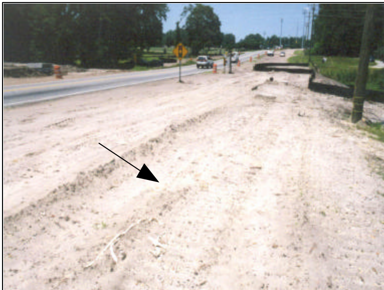
Photo 2. Incident job site and approximate location of incident (arrow)
