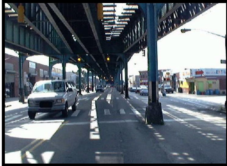
Photo 2. Northern approach to crash site showing track support columns (source, National Automotive Sampling System)
