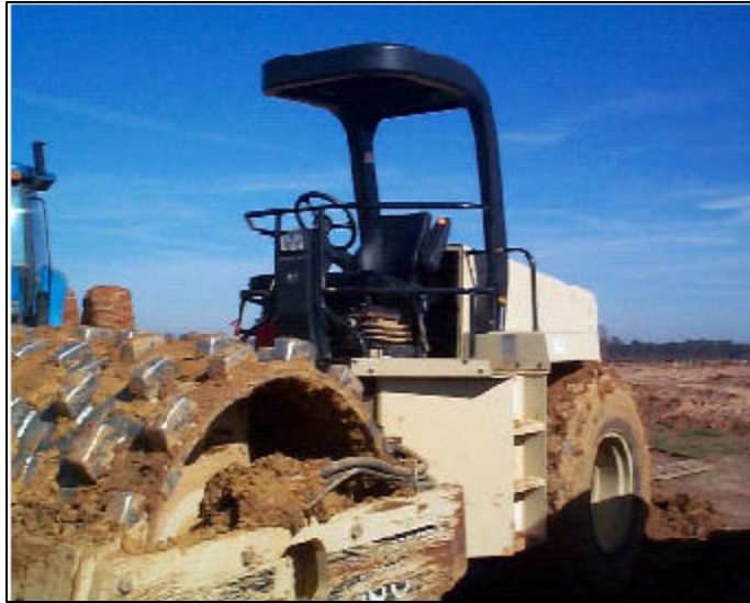
Photo 1. Compactor involved in the incident
