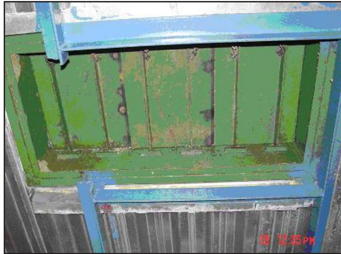
Photo 8. Overhead entry portal with cover in place.
