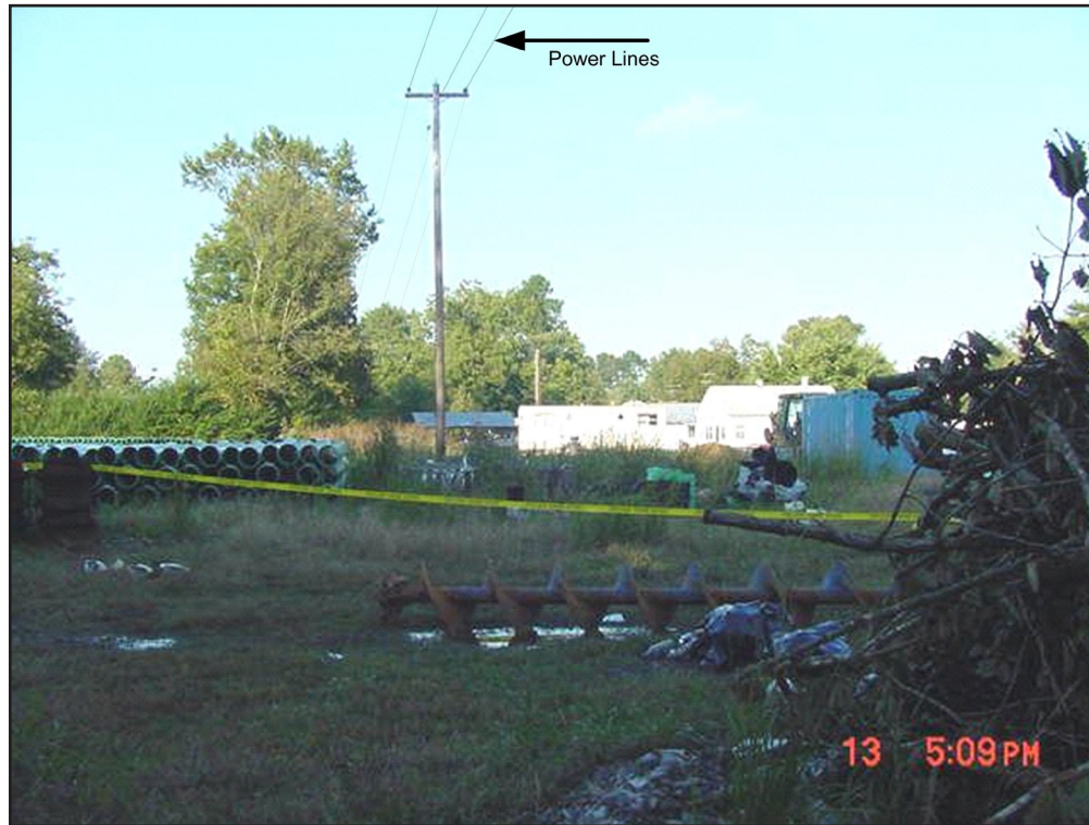
Photo 2. This photo illustrates the overhead power lines located at the materials storage yard. [Photograph courtesy of NCOSH].
