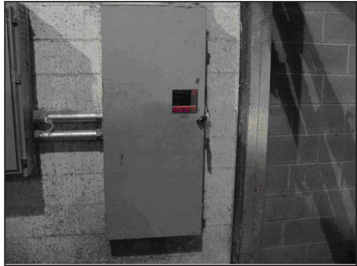
Photo 3. This photo illustrates the energy source to the Densifier which was de-energized and locked out before EMS personnel entered the Densifier to remove the victim's remains [Photograph courtesy of TDLWD].
