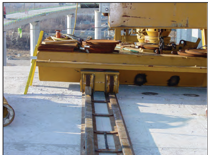
Photo 5. Close-up showing roller beam resting on track.
