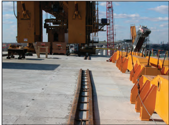
Photo 4. View of the railway system behind launching gantry LGL.
