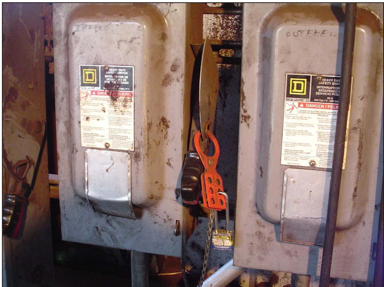
Photo 2: This photo illustrates the south debarker room where locks had been placed on two electrical circuits by the victim [Photo courtesy of SCOSHA].
